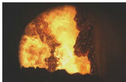
Blick in die Brennkammer
